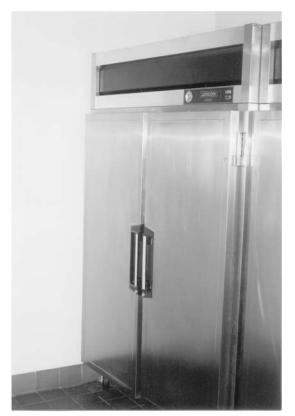
A reach-in refrigerator is used for storage of prepared food prior to service
